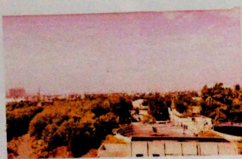
Koyambedu Sewage Treatment Plant Sewage treatment plant
